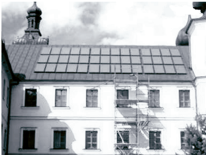
Fig. 1. South oriented solar collectors on a roof at the Cloister of Redemptorists, Tuchow, Poland
